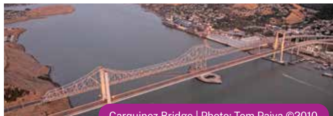
Carquinez Bridge | Photo: Tom Paiva ©2010
